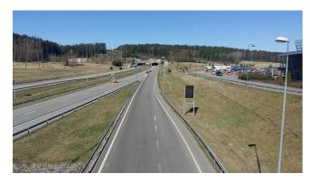
Caverion will execute a project to modernise a telematic system, installed in 2003, over a 60-kilometre stretch of motorway. Work began in May and the target is to deploy the new system by the end of the year. At the same time, the concrete and steel structures and ventilation system in the 435-meter-long lsokylä tunnel will be repaired and the tunnel's safety systems will be modernised. The tunnel works will continue until midsummer.
